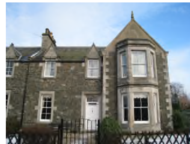
Figure 10: Eddleston Street Frontage
