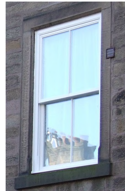
Figure 22: Acceptable Replacement Window
