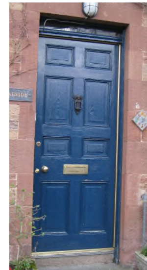
Figure 24: Example of a Panelled Main Entrance Door
