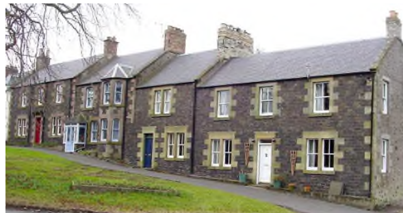
Figure 2: Historic Street Frontage - Yetholm
